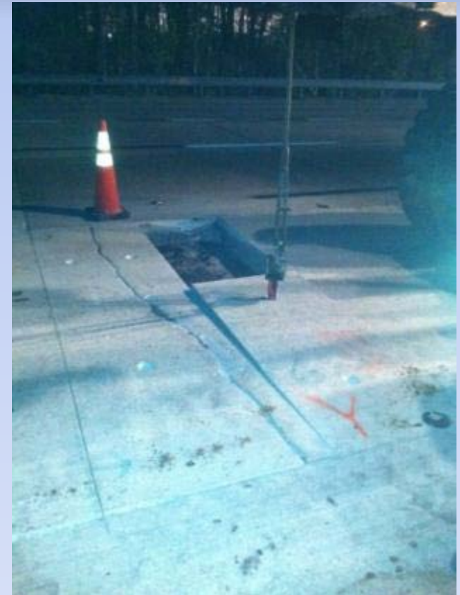
Slab Removal
